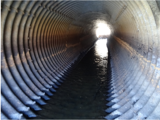
Picture 5: Culvert Barrel
