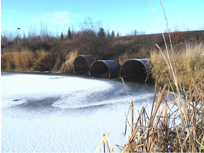
Picture 1: Culvert Inlet
