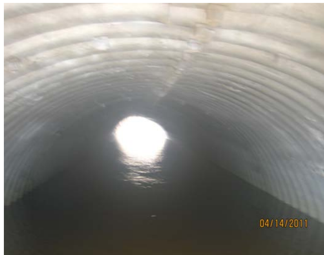
CMP05 - Outlet Barrel
