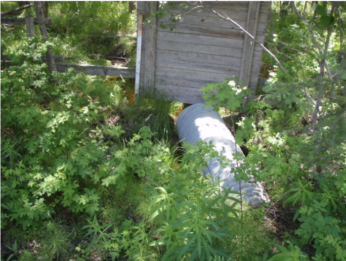
CMP25 – Inlet culvert barrel (South)
