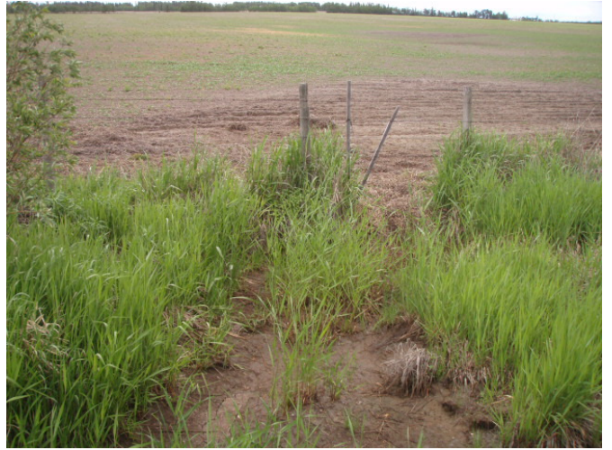
CMP15 – Inlet looking upstream (East)
