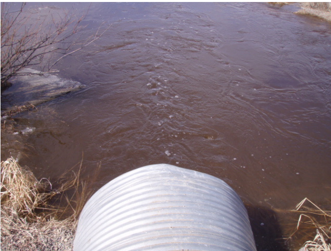
CMP (22-23) – Outlet Barrel
