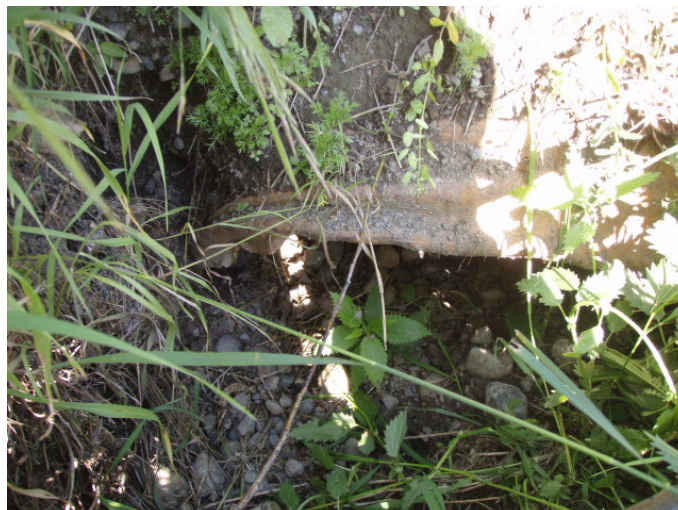
Private CMP07 – Outlet looking (West)
