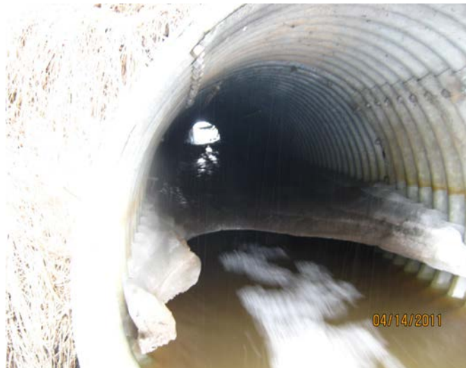
CMP (02-03) – Outlet Barrel
