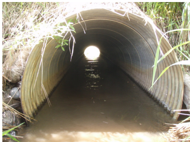
CMP (06-07) - Inlet Barrel
