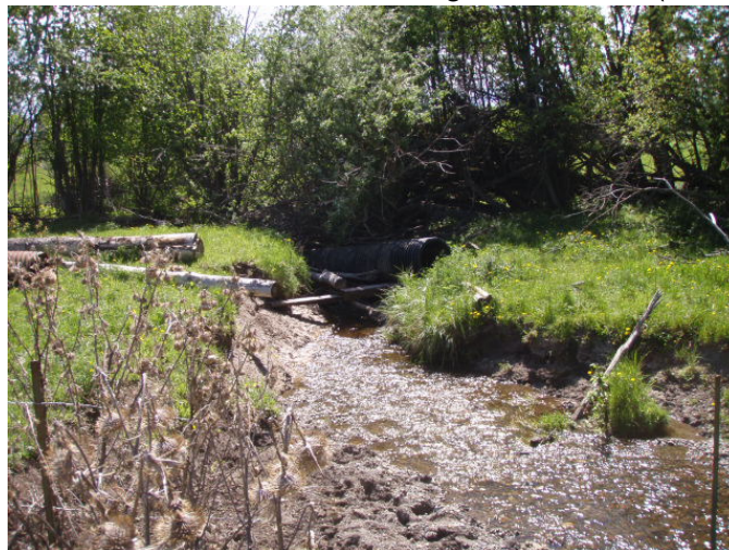
Private CMP06 – Outlet looking downstream (South)
