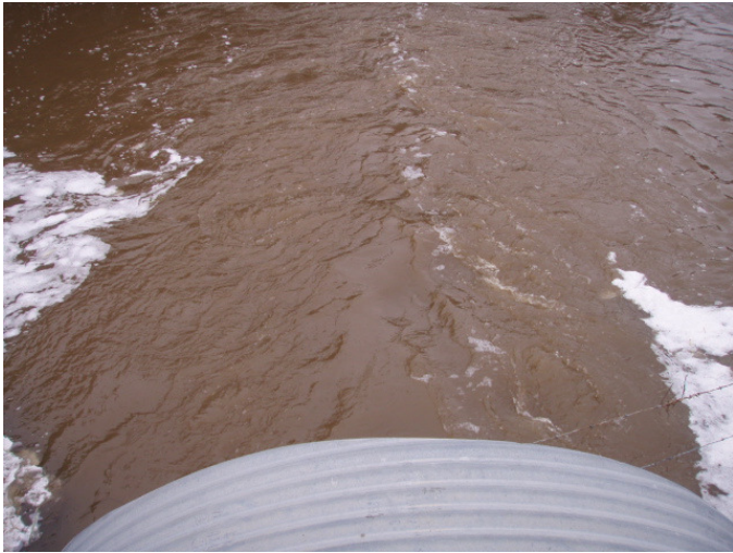
CMP11 – Outlet Barrel
