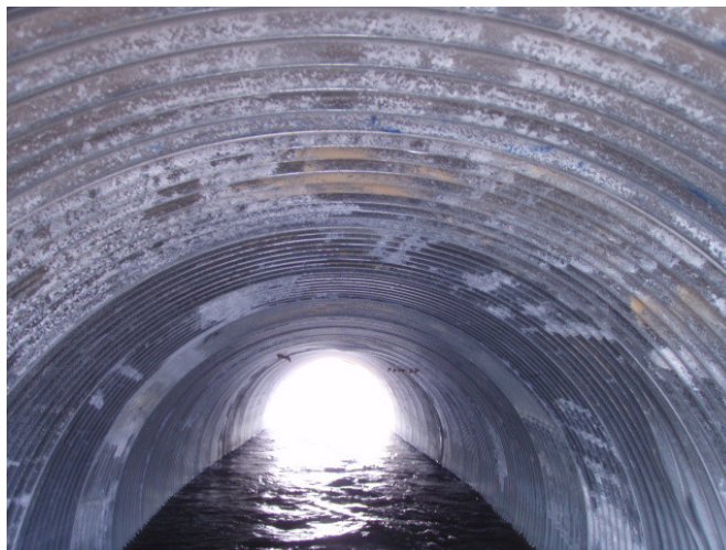
CMP (22-23) – Outlet Barrel
