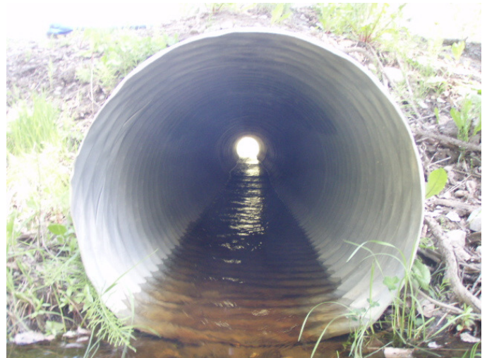
CMP19 – Outlet Barrel
