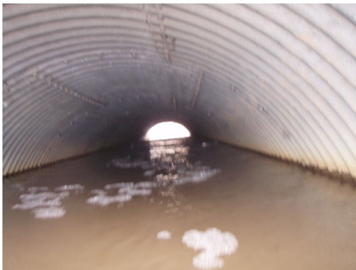
CMP12 – Outlet Barrel
