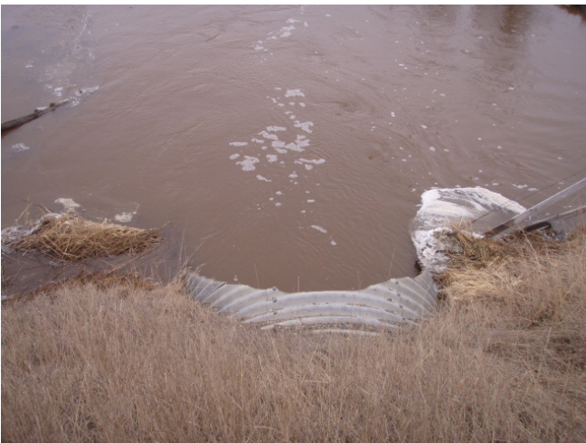
CMP12 – Outlet Barrel
