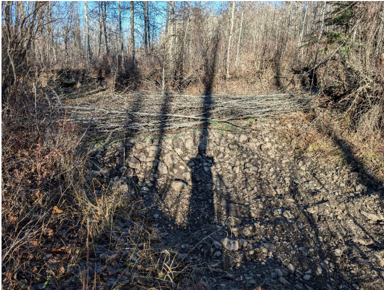
Figure 7: Completed BDA without posts
