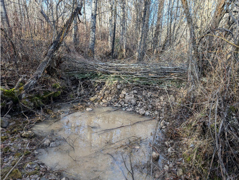
Figure 8: Completed BDA without posts
