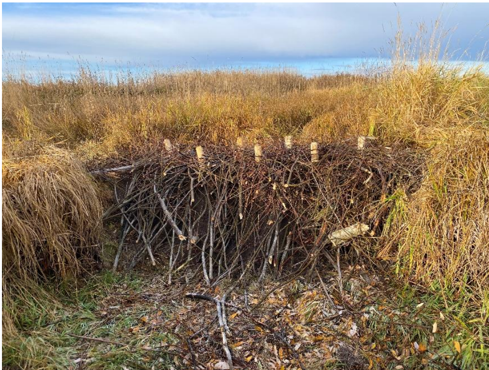
Completed BDA in-stream.
