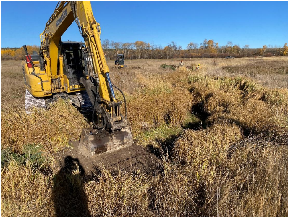
Photo of excavator operating from above the stream bank while constructing a BDA.
