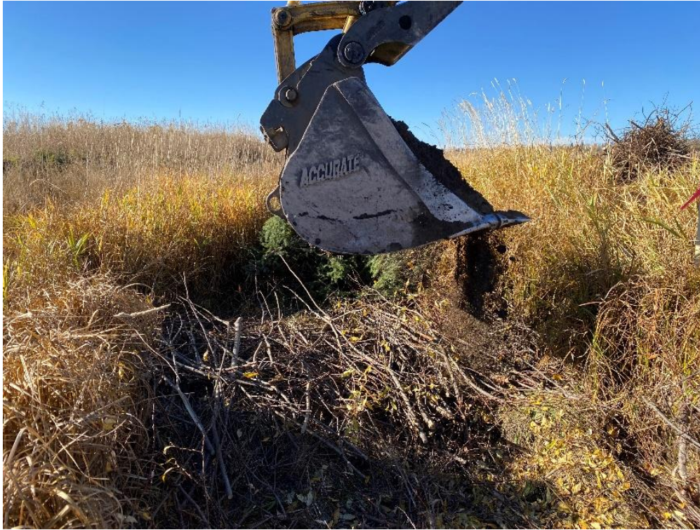
Building of BDA using backhoe.
