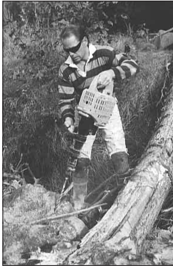
Figure 7-24b. Anchoring LWD structures.
