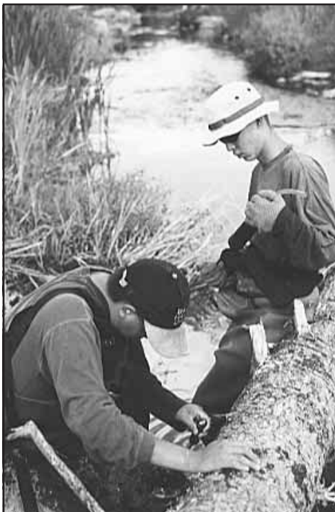
Figure 7-24a. Anchoring LWD structures.
