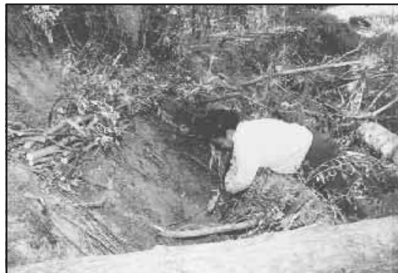
Figure 7-25. Willow wattle and brush layer placement.
