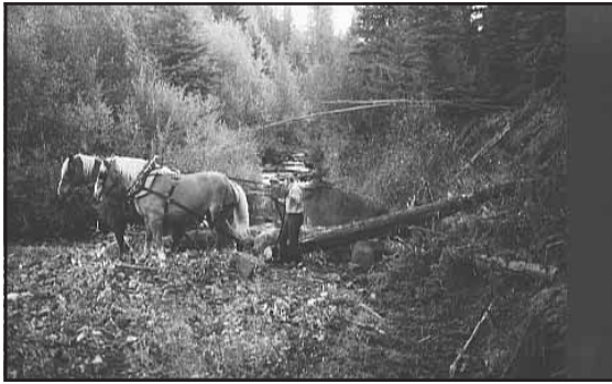
Figure 7-22. Draft horses placing LWD.
